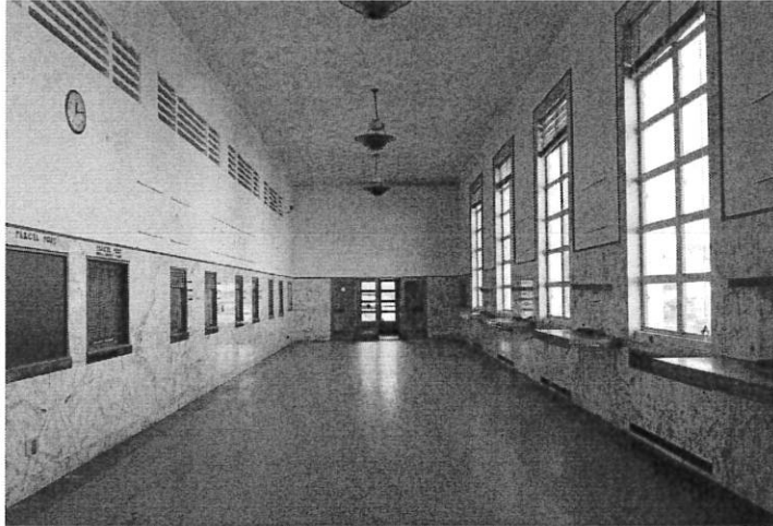
Figure 2: Lobby, looking towards the Park Road entrance.
