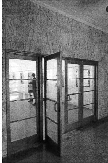
Figure 5: Vestibule doors to lobby.
