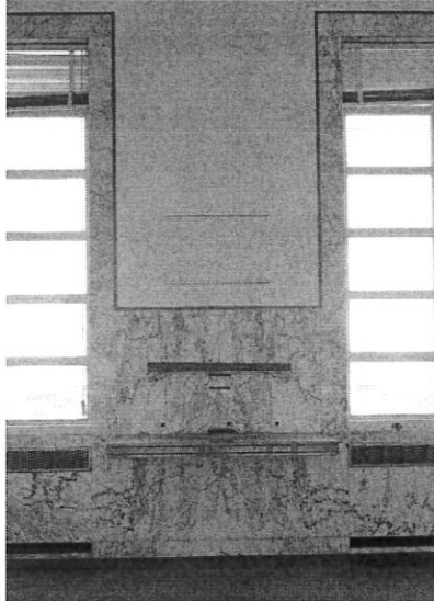
Figure 4: Cantilevered desks between lobby windows.
